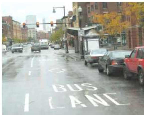
Source: TCRP Report 118 – BRT Practitioner’s Guide On-street bus lane (Silver Line, Boston)
