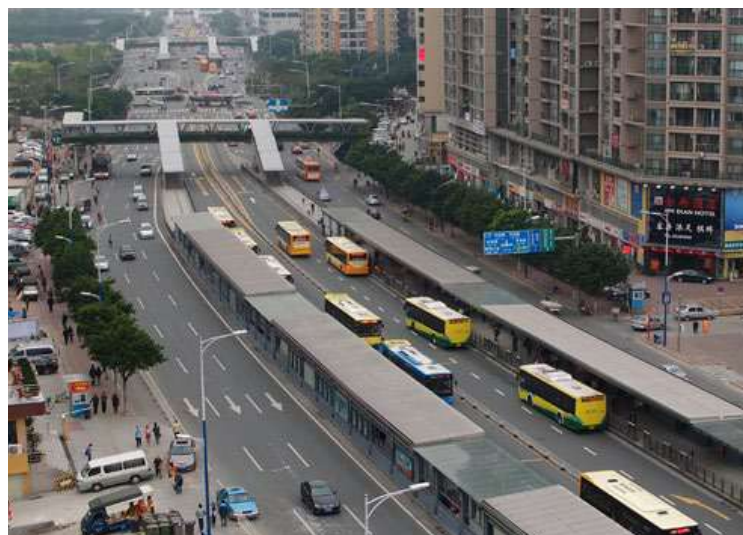
Figure 21 : Typical BRT station side platform
